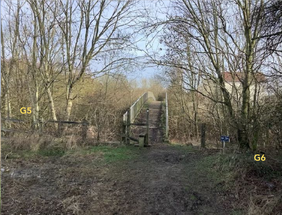
IMAGE 2: A view looking east at the PRow footbridge which crosses the A10
